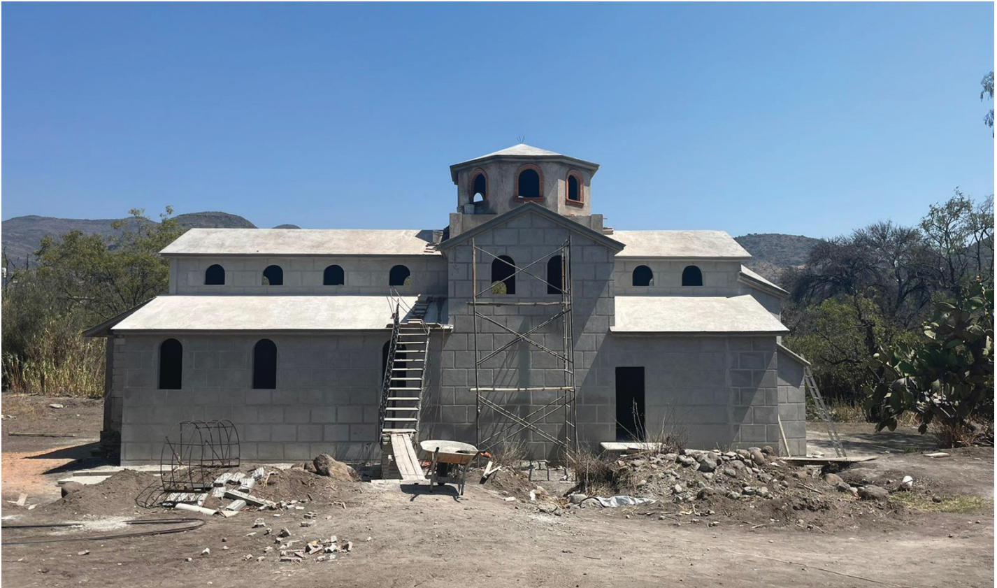
Chapel for San Basilio Orthodox Pastoral Academy under construction.
